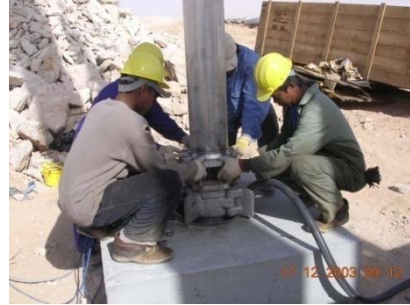
One of the numerous wells in the project is being established.
